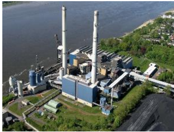
Wedel CHP plant, Germany
