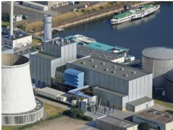
Köln-Niehl combined-cycle heat and power (CHP) plant in Cologne, Germany
